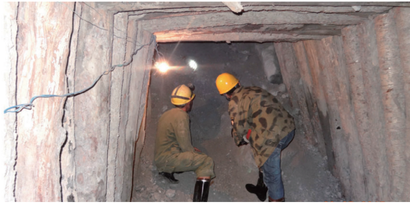
Figure 5-2: Existing Supporting Measures for A Main Passing through a fault zone
