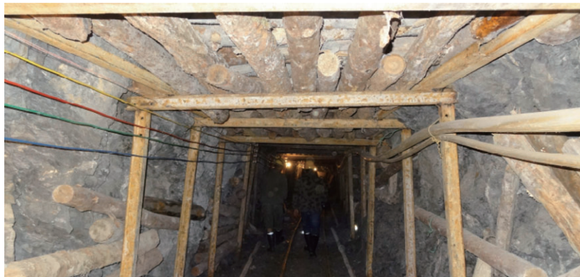
Figure 5-2: Existing Supporting Measures for A Main Passing through a fault zone
